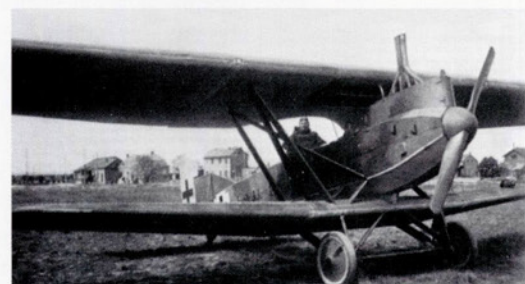
The Junkers J 1 (factory designation J 4) entered service in the Infanterieflieger units in 1917. The aircrews viewed the aircraft with considerable favour, due to it being immensely strong and also for the armour protection it afforded. The machine was used to fly low over the trenches and supply troops with ammunition and rations as well as low-level machine gunning of enemy trenches.
